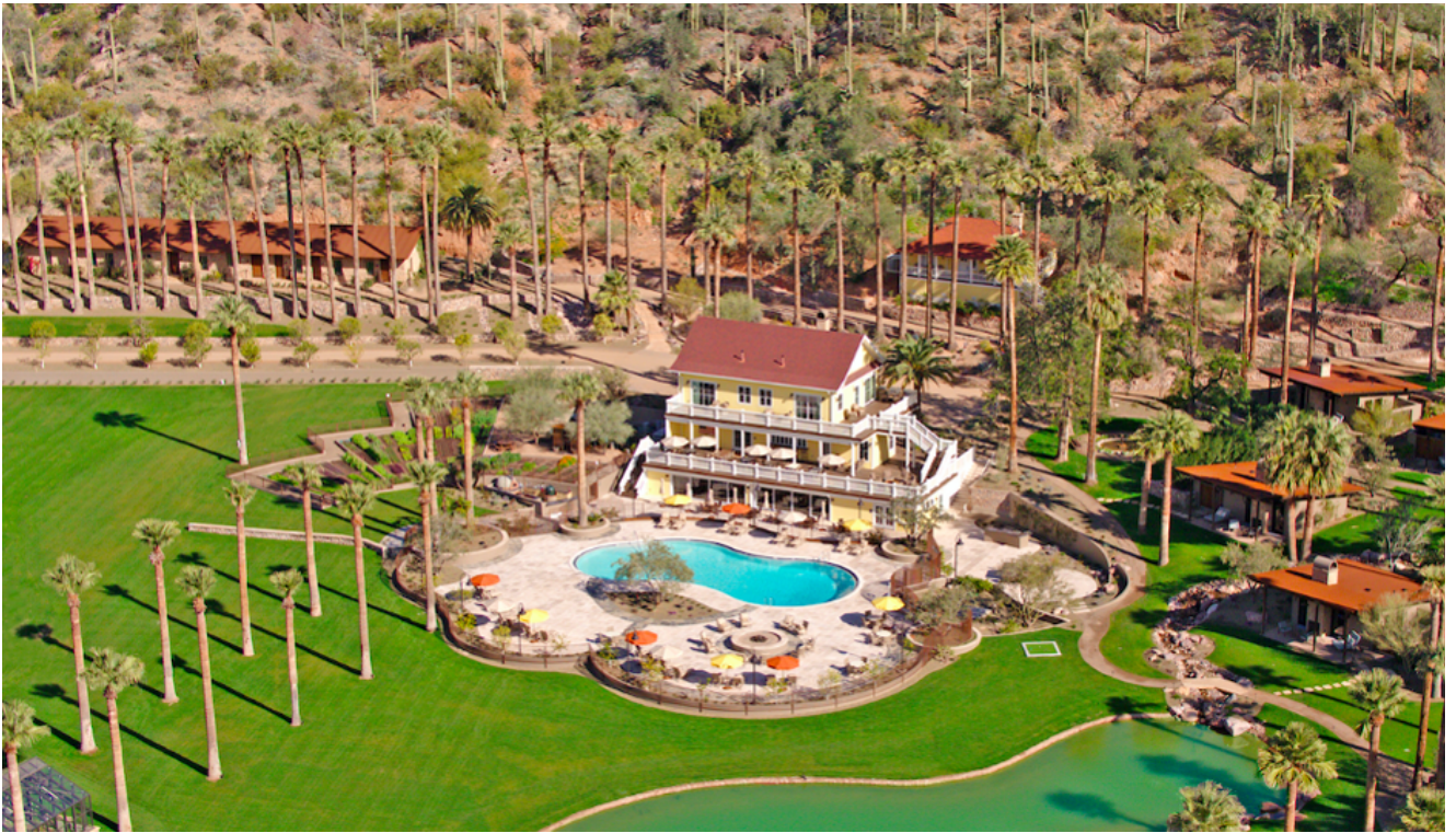
An aerial view of Castle Hot Springs' main lodge. PHOTO COURTESY OF CASTLE HOT SPRINGS
